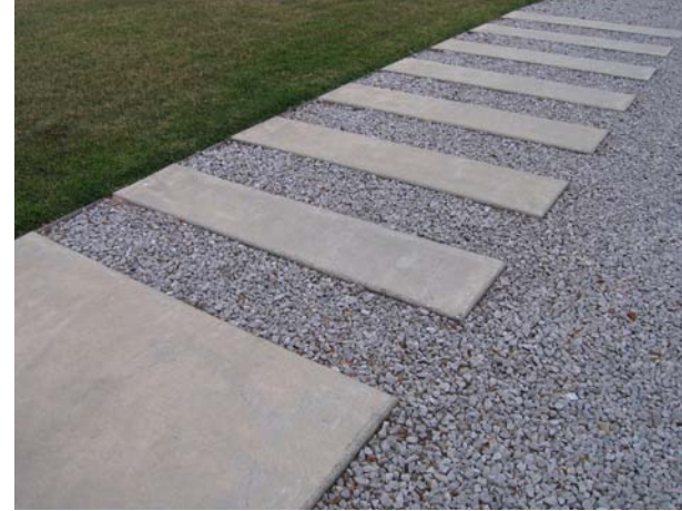
water permeable driveway
